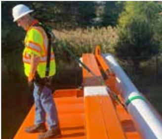
Designed to be used as a personal anchor for human support. This Buck anchor strap with a wear guard has a choking configuration and is small, lightweight, and flexible making it easy to handle and install in the field.
