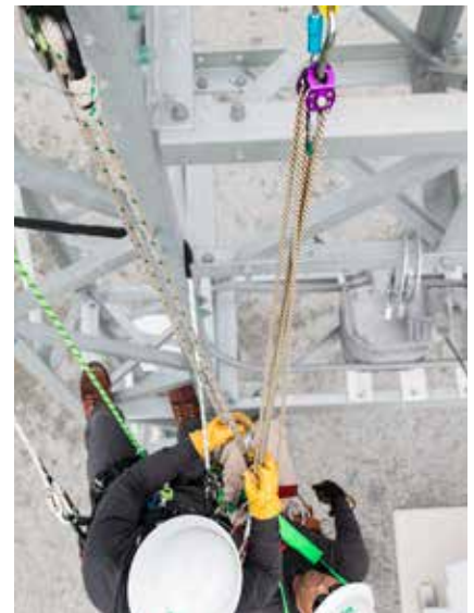
3. Rescue, lowering with the OX BLOCK™.
