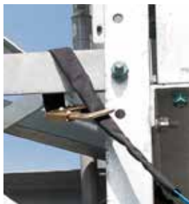
Close up of tie-back snap with wear guard.
