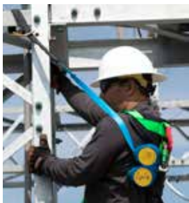
Using Dual Tie Back BuckLimiter™ with the BuckArticulator™ harness.
