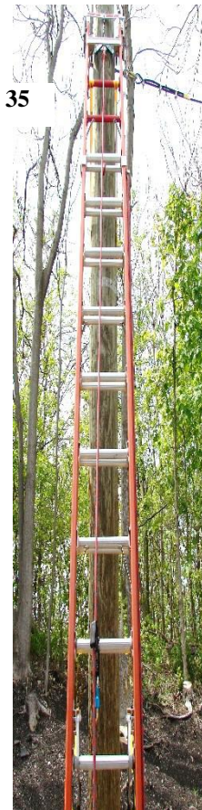
Pole Properly Seated in V-Rung / V-Bar
