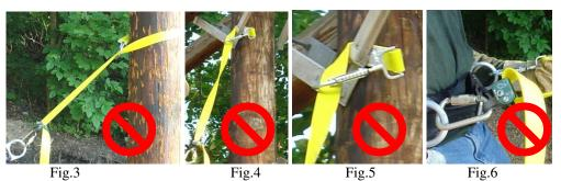
Examples of Improper Attachment (Ref. Fig. 3 - 6):
